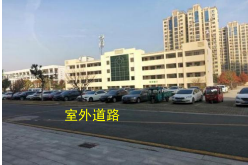
图 8-5 DSA 机房拟建址北侧
